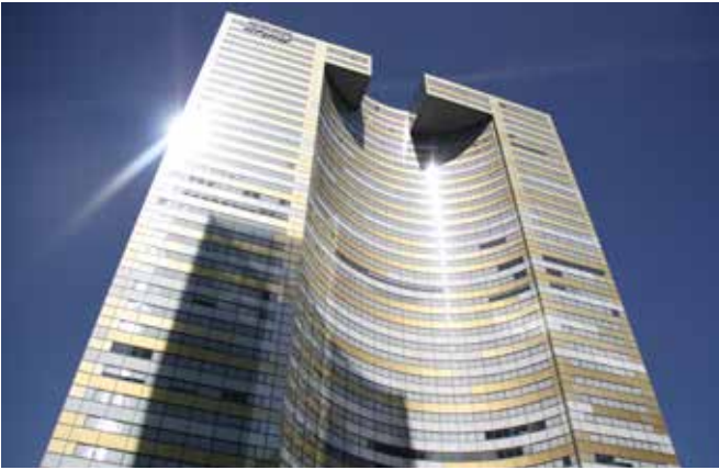
Tour Eqho - France - Clima Canal
